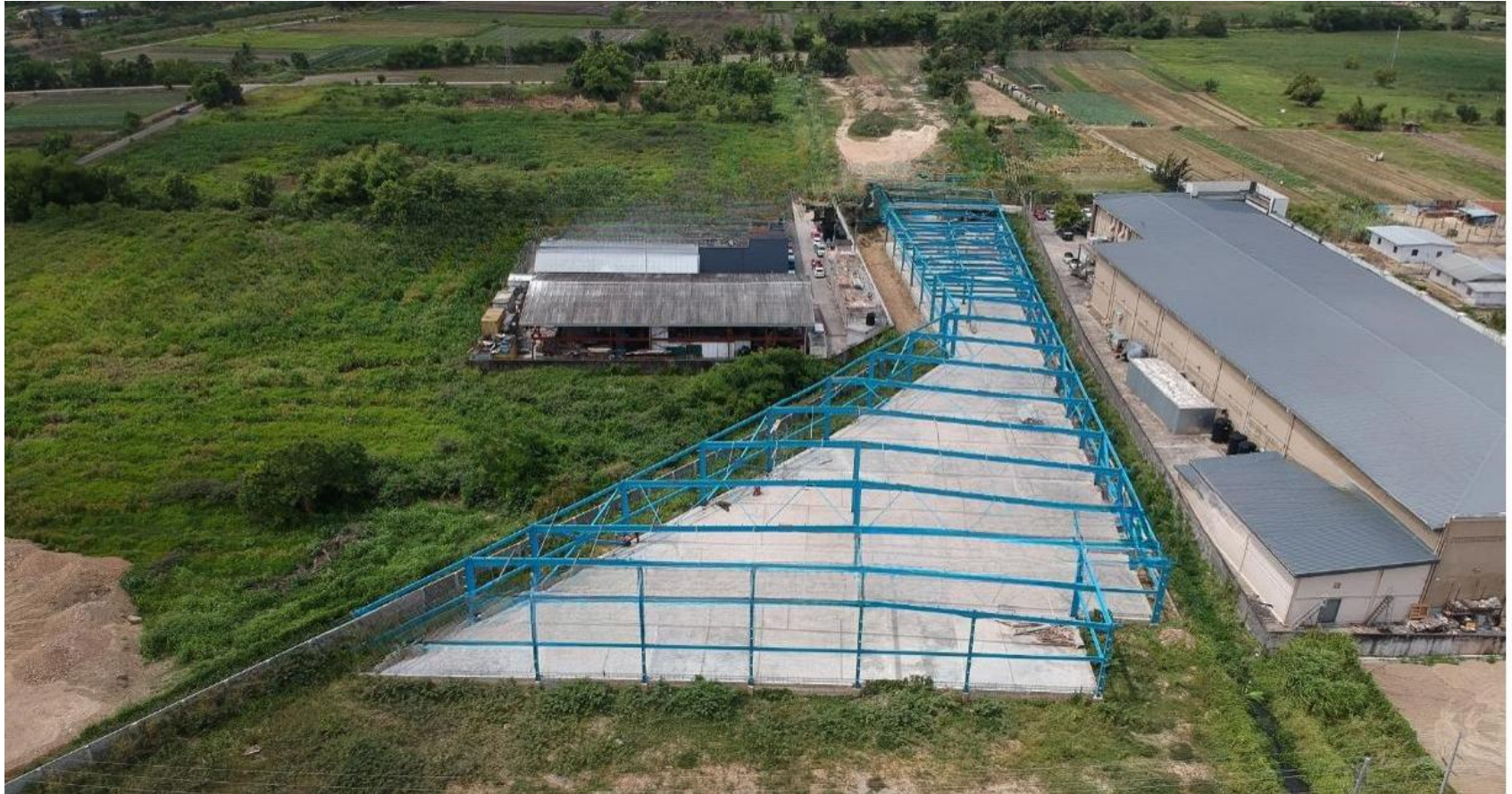
Steel Structure Building in Trinidad & Tobago Area: 3,000 sqm
