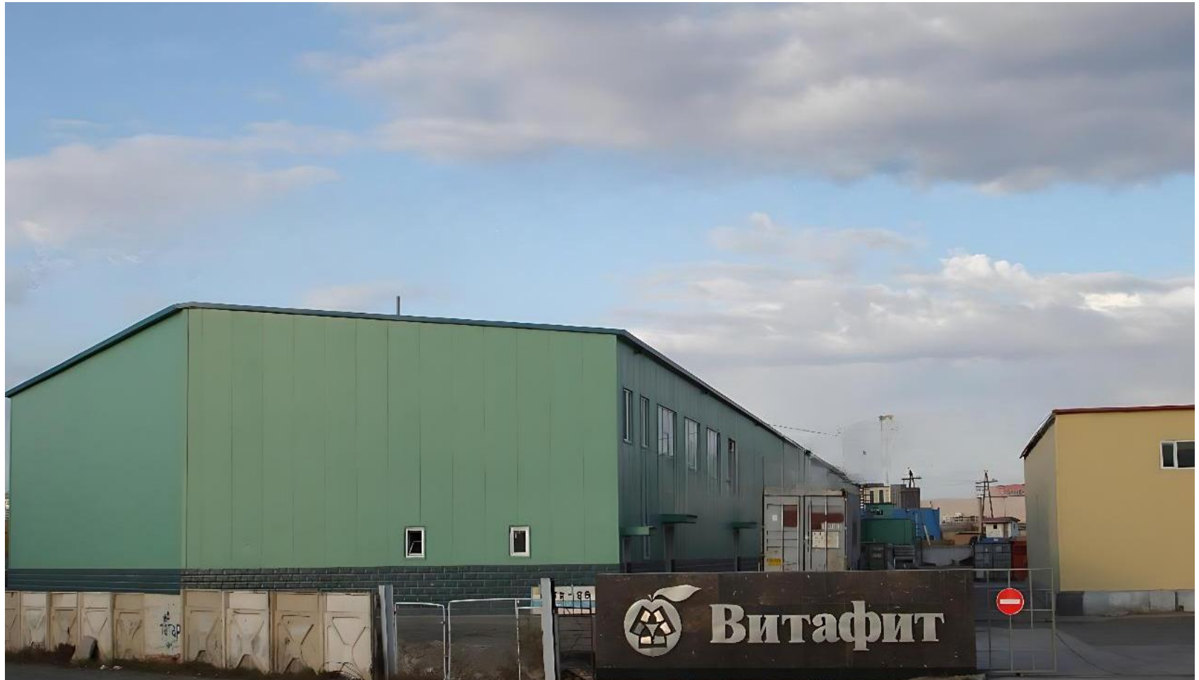
VIFAFIT in Mongolia, beverage manufacturing plant, 100mm green PU wall panels, 2,500 sqm
