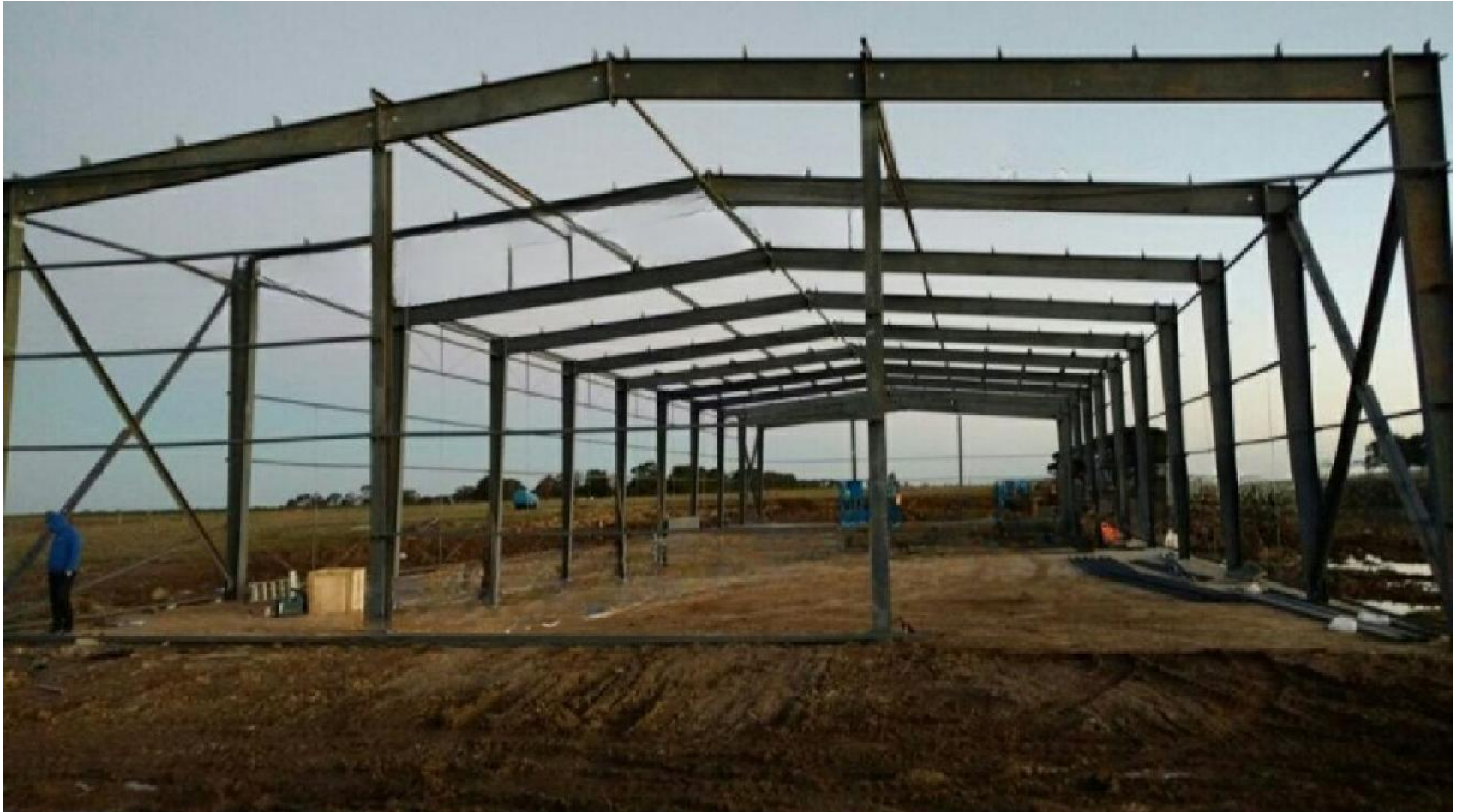
Workshop Project in Australia Area: 2,000 sqm
