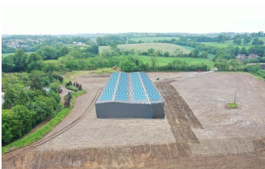
Factory project in UK Area: 3,500 m 2 with PU wall and roof sandwich panel
