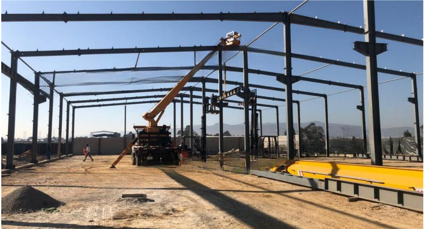
Workshop with Overhead Crane in Mexico Area: 75*30*7m
